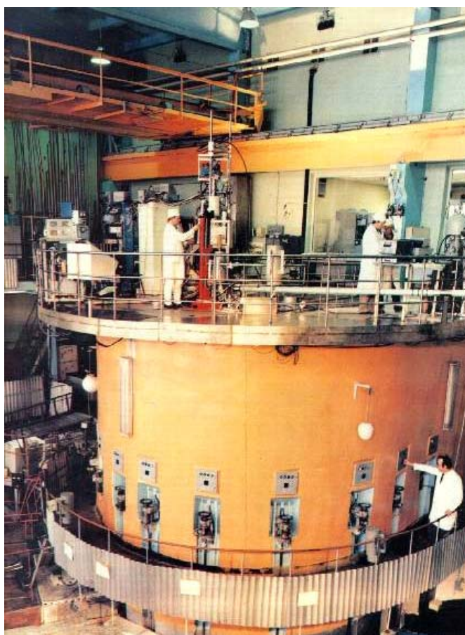
Fig. 1. MEPHI reactor: a 2.5 MW water-moderated pool-type reactor with a beryllium-water reflector, with 10 horizontal and 20 vertical channels. Thermal neutron flux in the reflector is 4.0 \times 10^{13} n/cm 2 /s.
