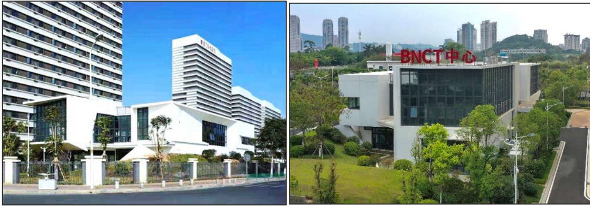
FIG. III-1. Xiamen Humanity Hospital BNCT centre.
