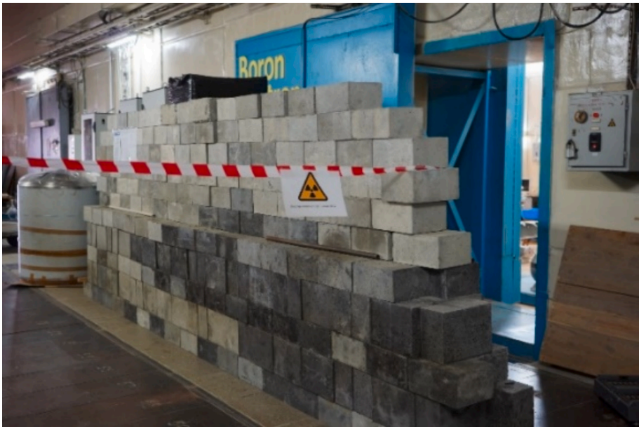
Fig. 6. Photo of the outside view of the bunker. This neutron protection wall contains boron for neutron capture to decrease neutron dose rate outside the bunker.
